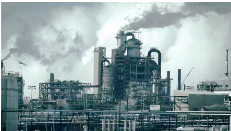
Figure 2. Fort McMurray's petrochemical plant
